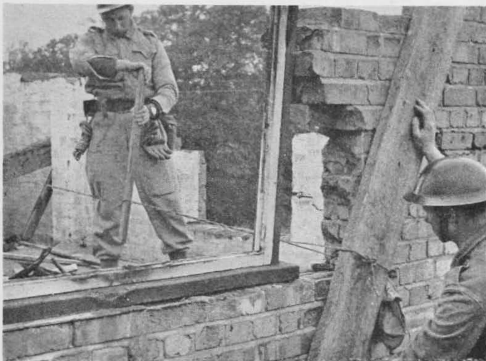
Fig. 22. Horizontal support of unsafe wall
