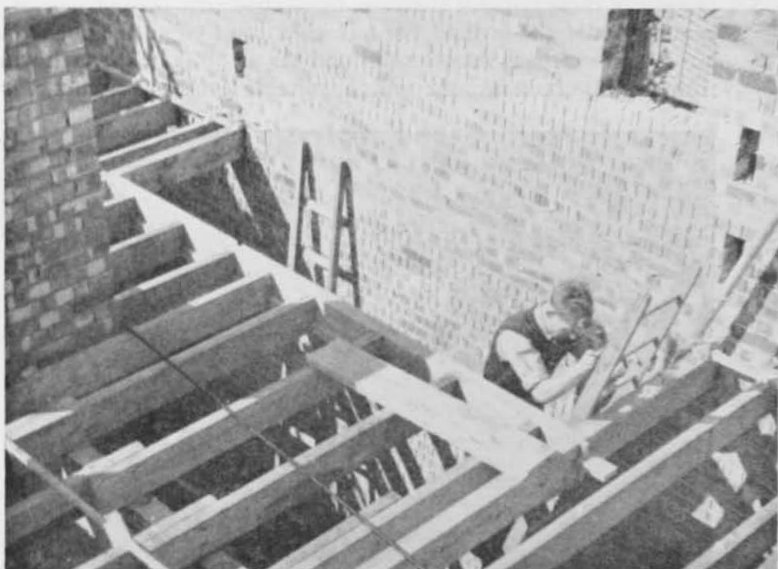
Fig. 14. Upper floor joists trimmed for staircase
