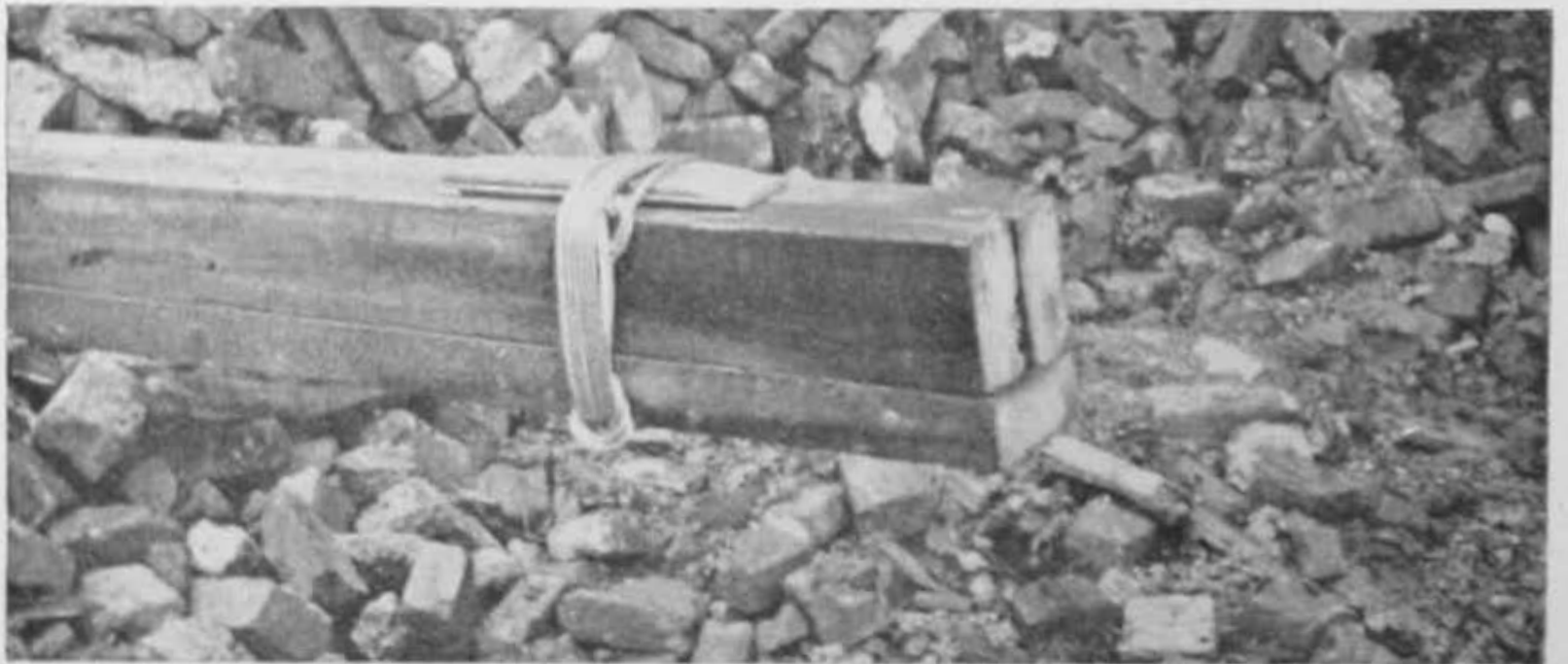
Fig. 18. Securing laminated timbers
