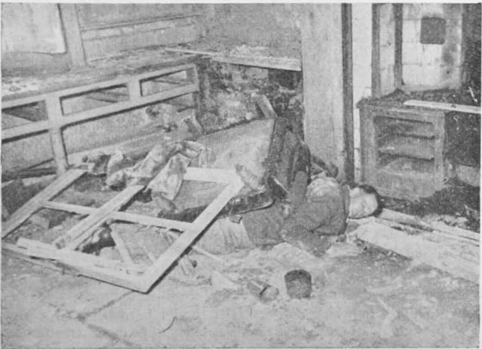
Fig. 141. Interior of slightly damaged building showing lightly trapped casualty
