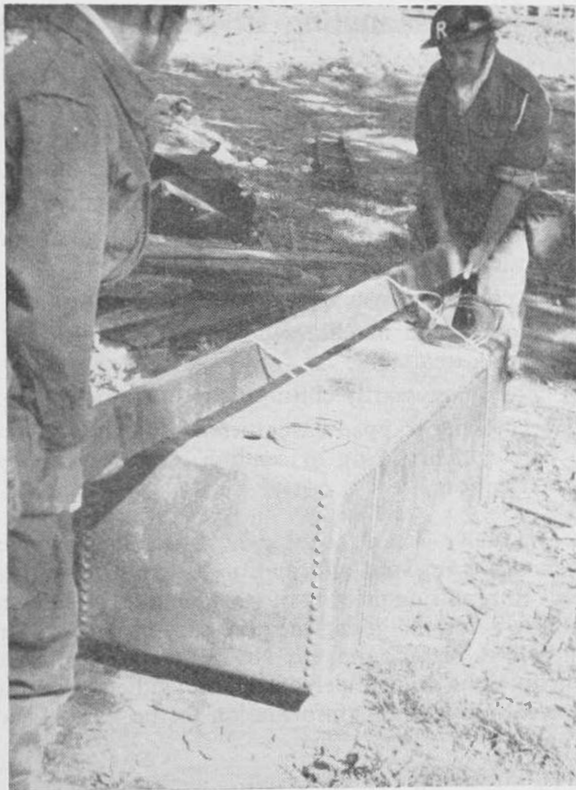
Fig. 25. Sling in applying direct lift
