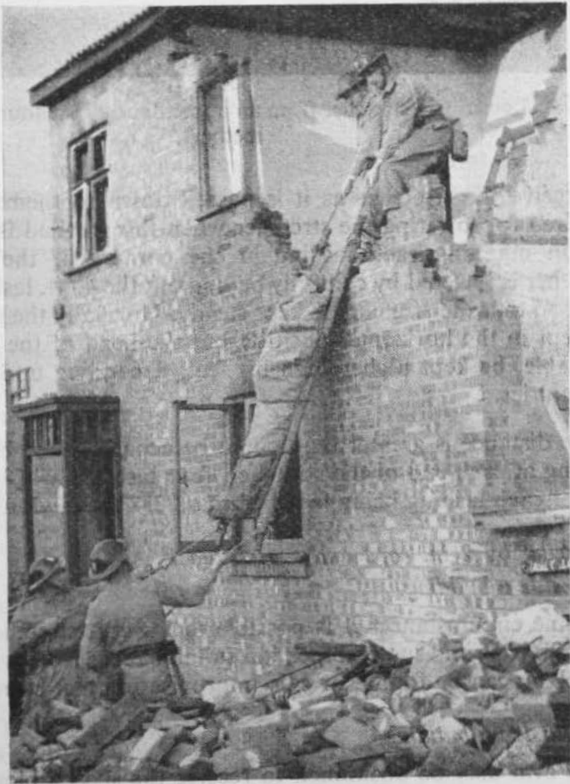
Fig. 97. Lowering a stretcher from an upper floor by two-point suspension method
