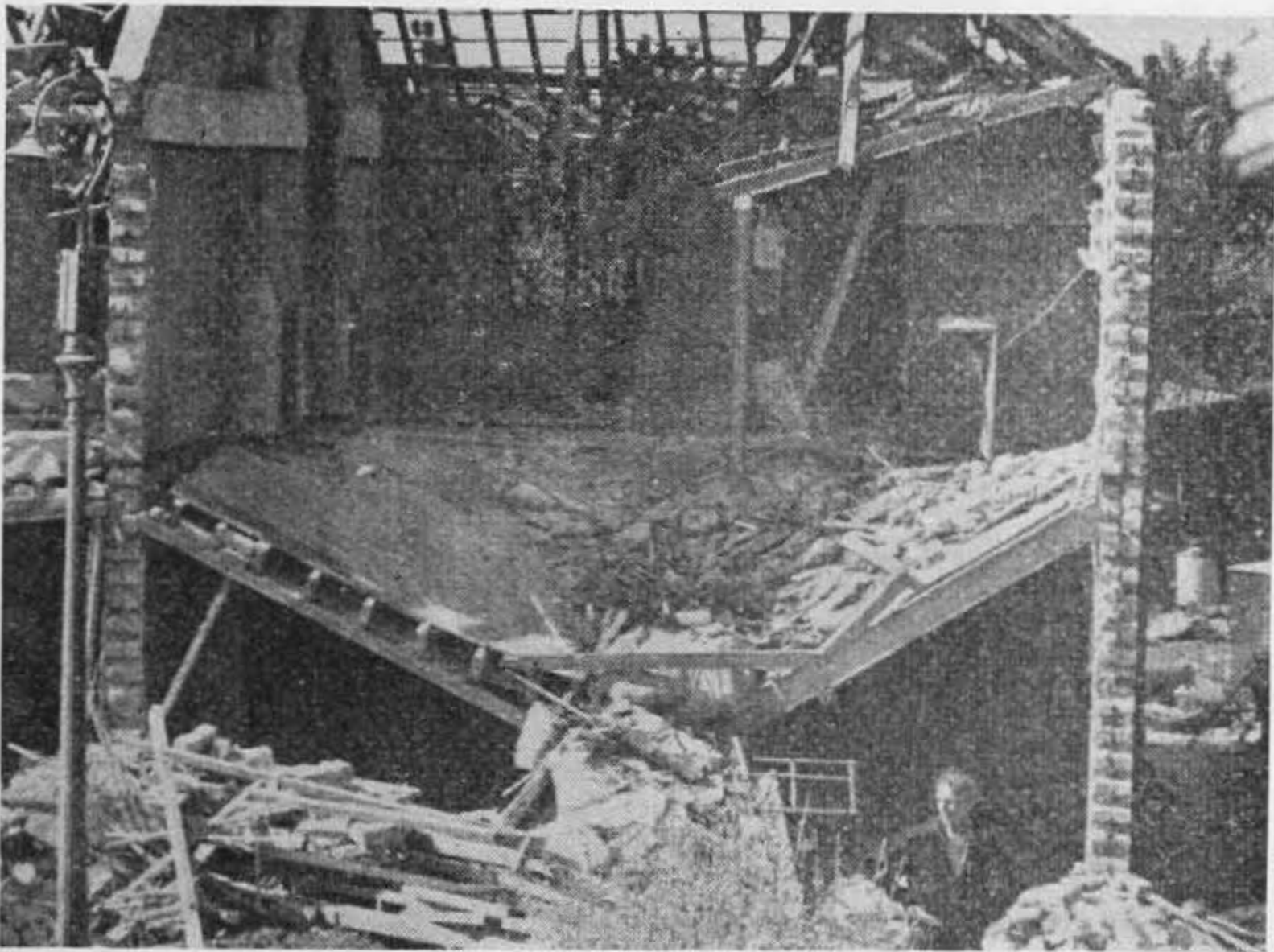
Fig. 78. Example of "V" form collapse (not in basement)
