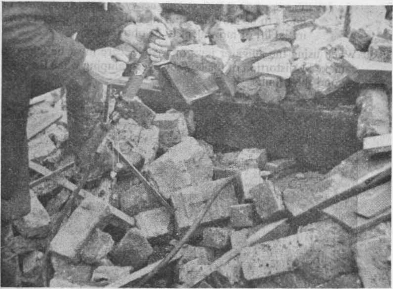
Fig. 123. The wedgie spreader being inserted under collapsed timber
