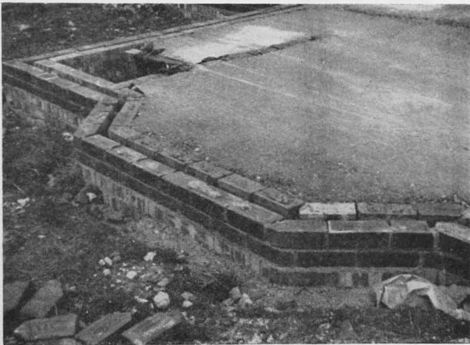
Fig. 13. Hollow walls built to damp proof course level
