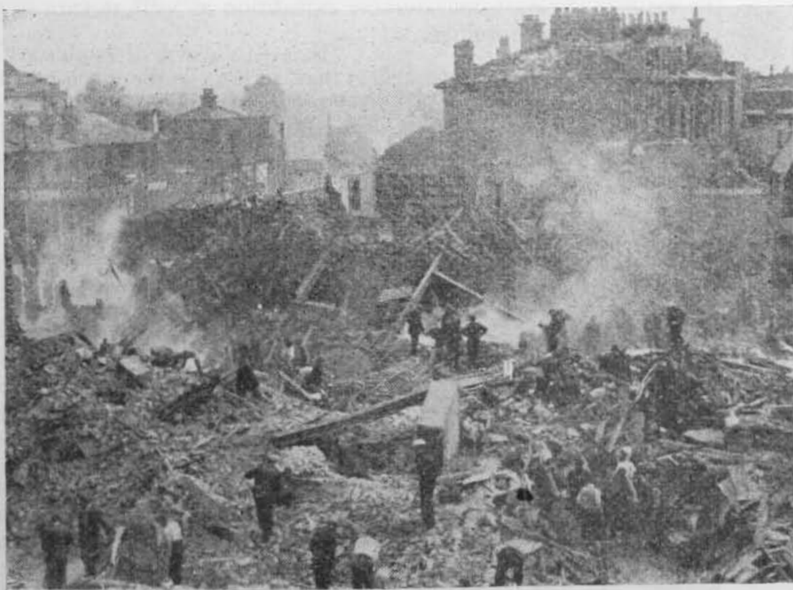
Fig. 81. Debris of buildings
