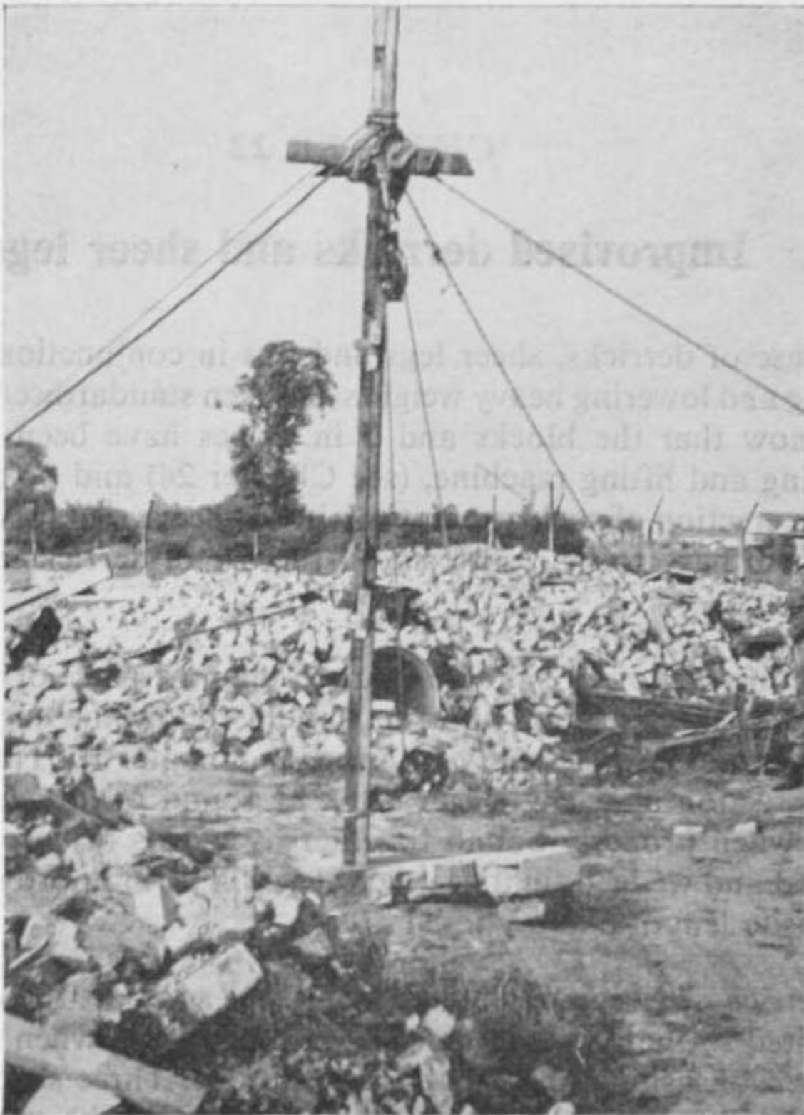
Fig. 90. An improvised derrick
