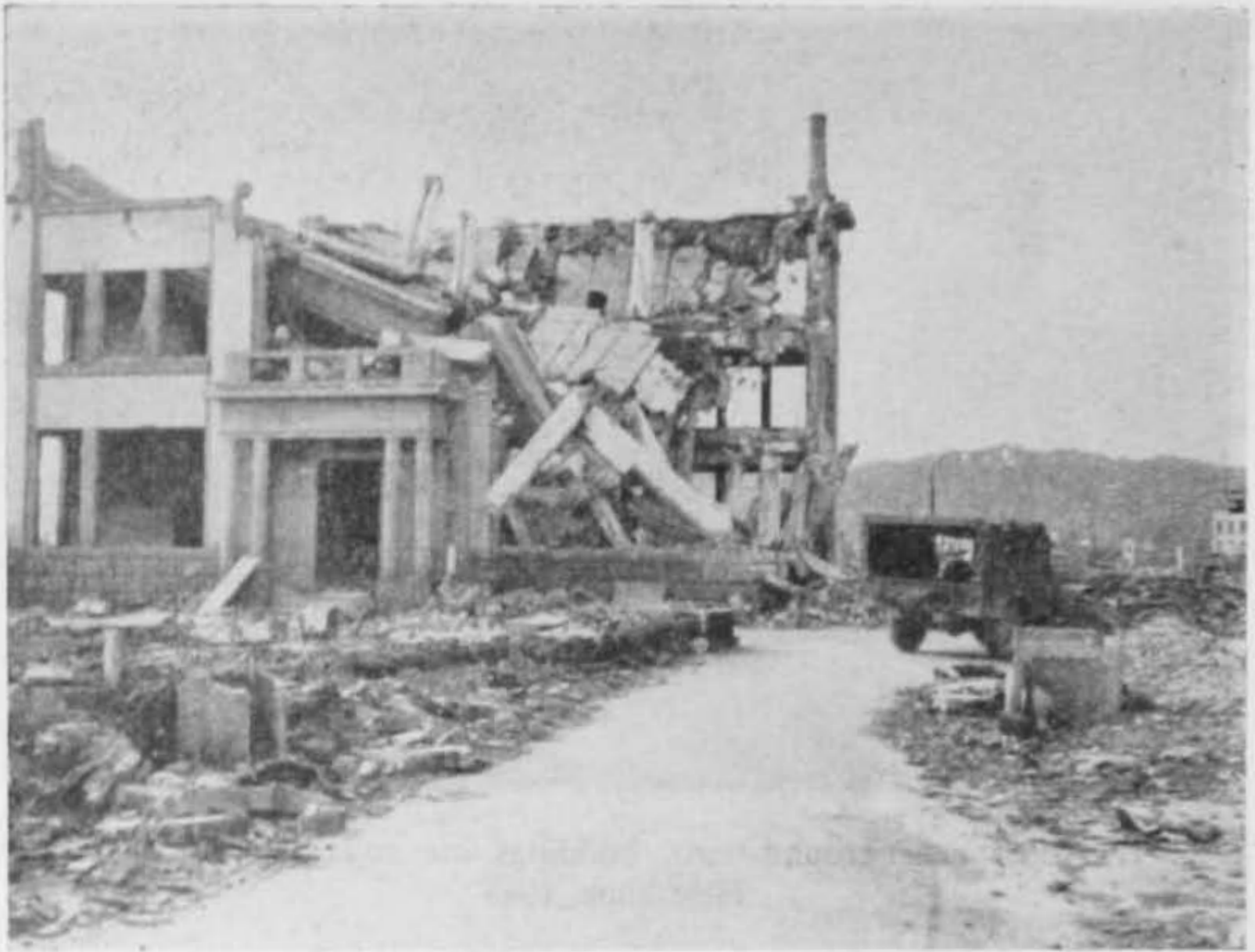
Fig. 3. With specially strong buildings, roofs are crushed or dished in, even while the walls remain standing : Hiroshima, 1945
