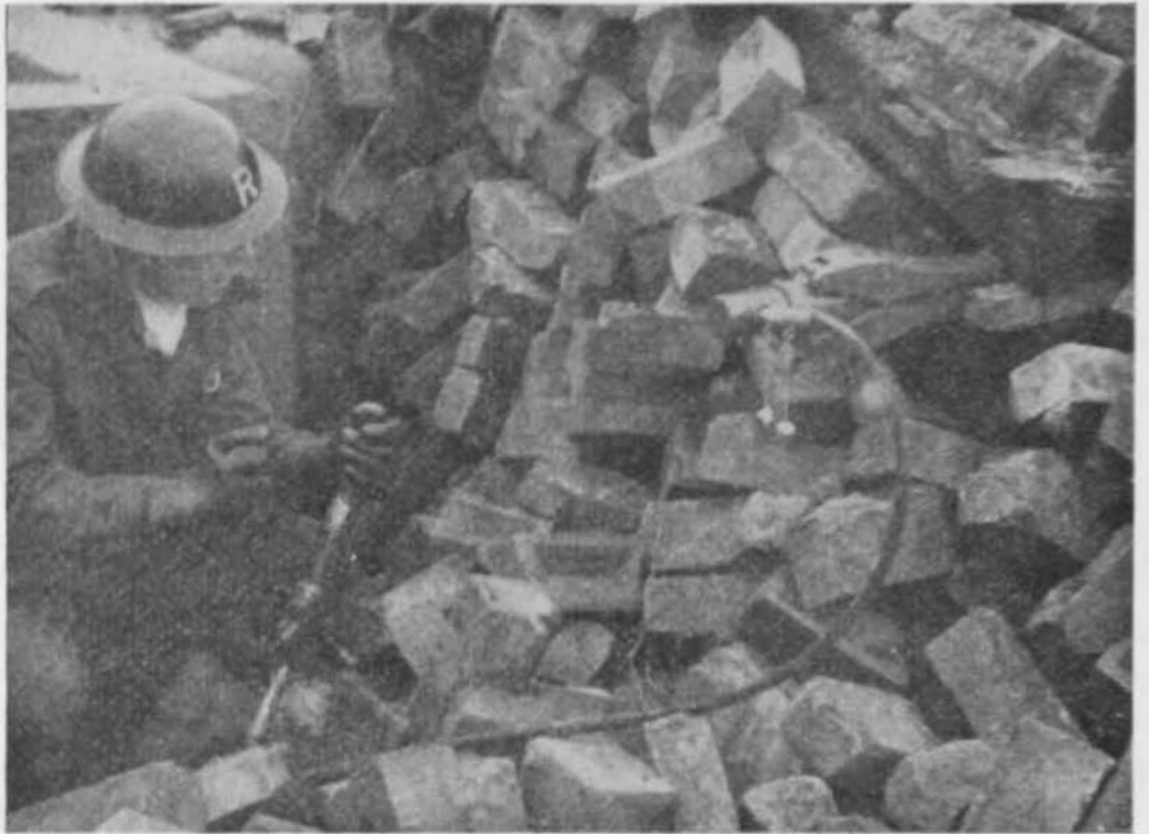
Fig. 122 (a). Another use of the alligator spreader
