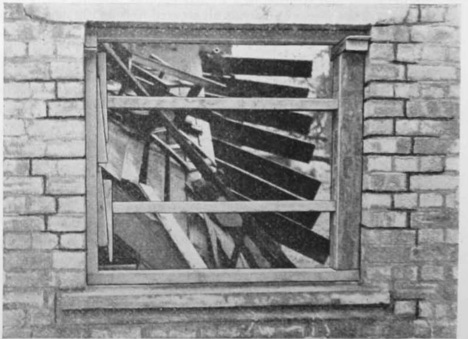
Fig. 69 (b). Strutting of window opening
