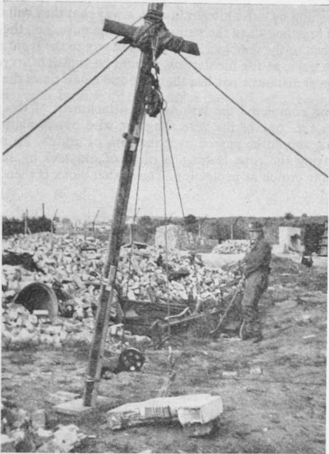
Fig. 92. Luffing a derrick
