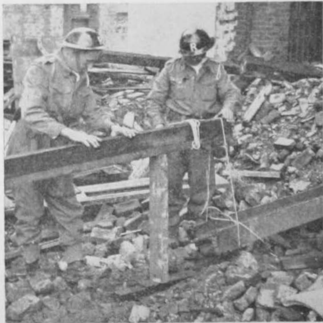
Fig. 24. Another wire bond sling in conjunction with a spar
