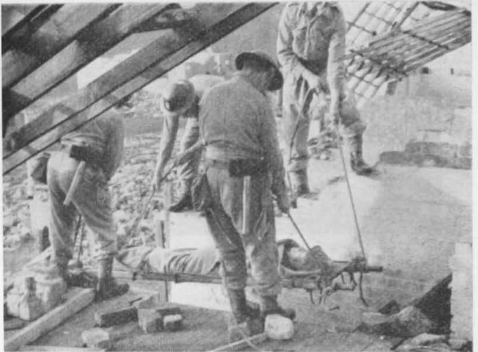
Fig. 98. Lowering a stretcher from an upper floor by the four point suspension method
