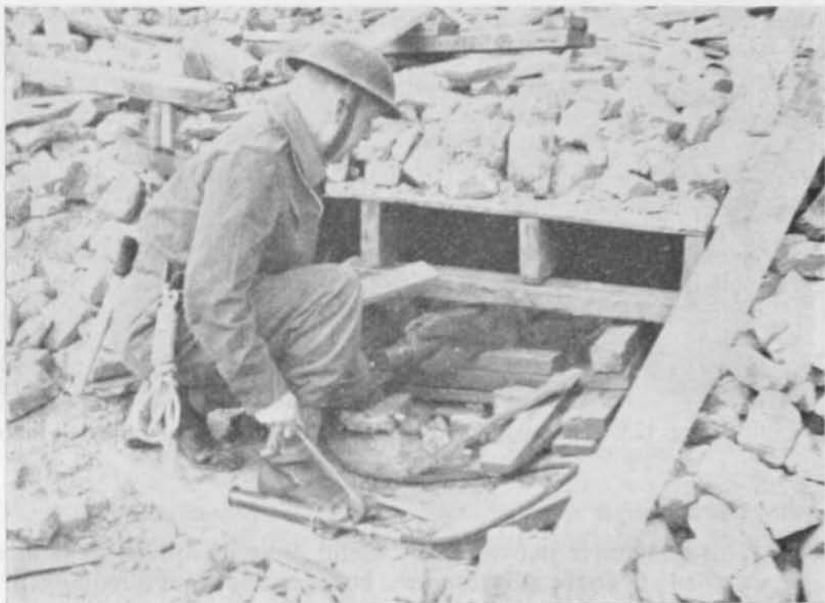
Fig. 124. The apparatus can be operated in a confined space by one man, who can pump with one hand and insert packing as required with the other.
