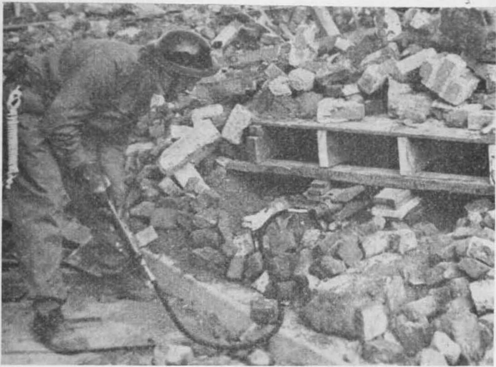
Fig. 120. Initial lift by the alligator spreader
