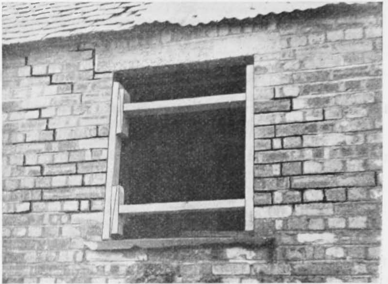
Fig. 69 (a). Strutting of window opening
