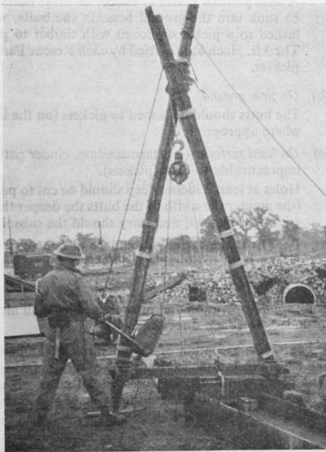
Fig. 94. Sheer legs erected, load being lifted by hauling and lifting machine
