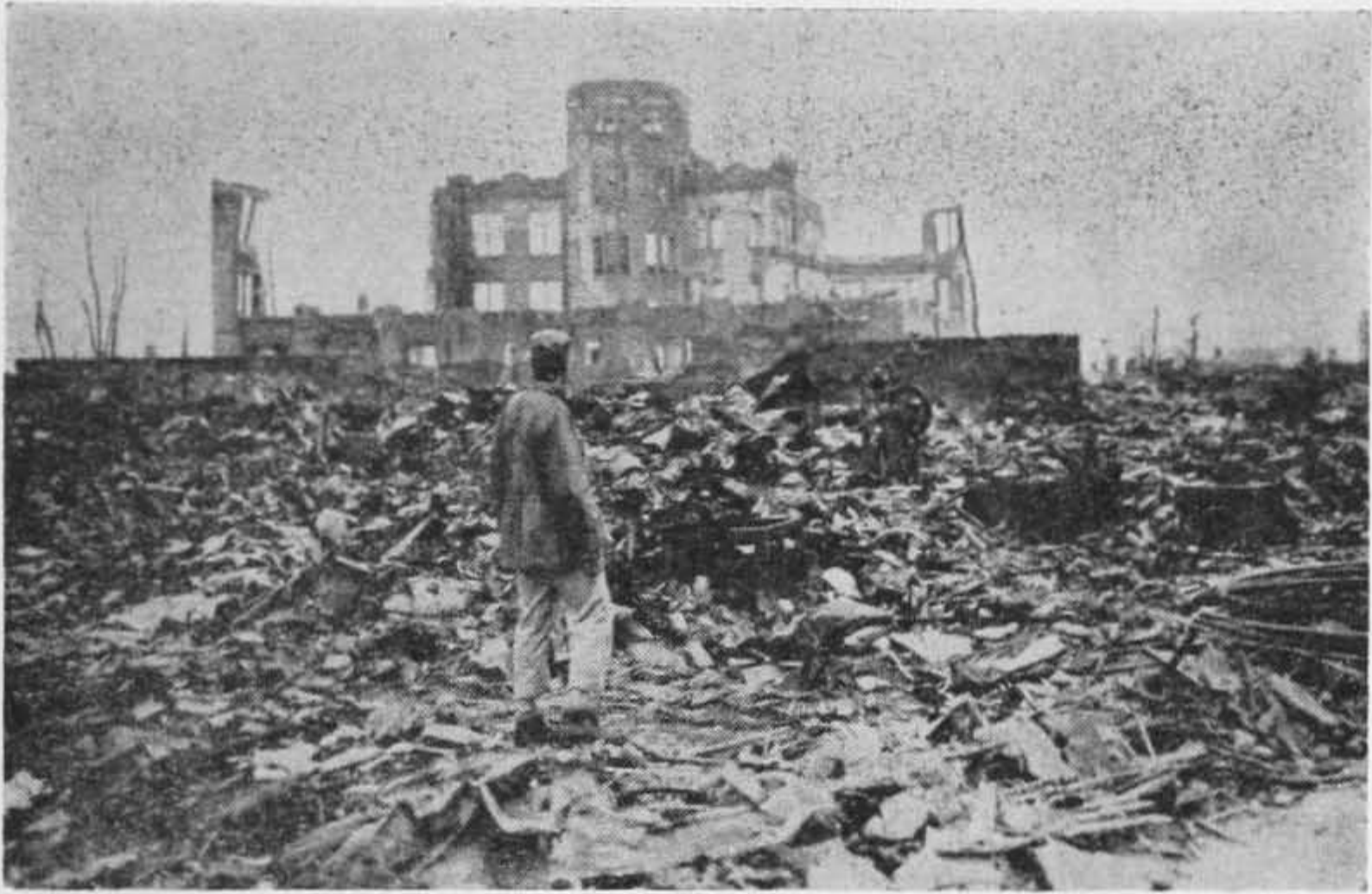
Fig. 1. At or near ground zero, buildings are collapsed on themselves: Hiroshima, 1945
