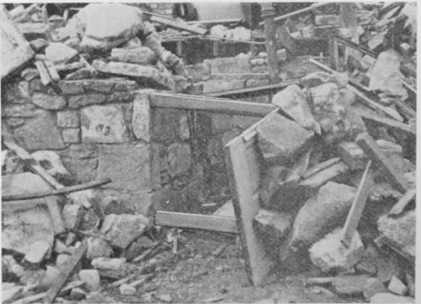
Fig. 72. Utilising an old door, struttled back from the remains of a stone wall, to hold up debris and form a crawlway for the extrication of casualties
