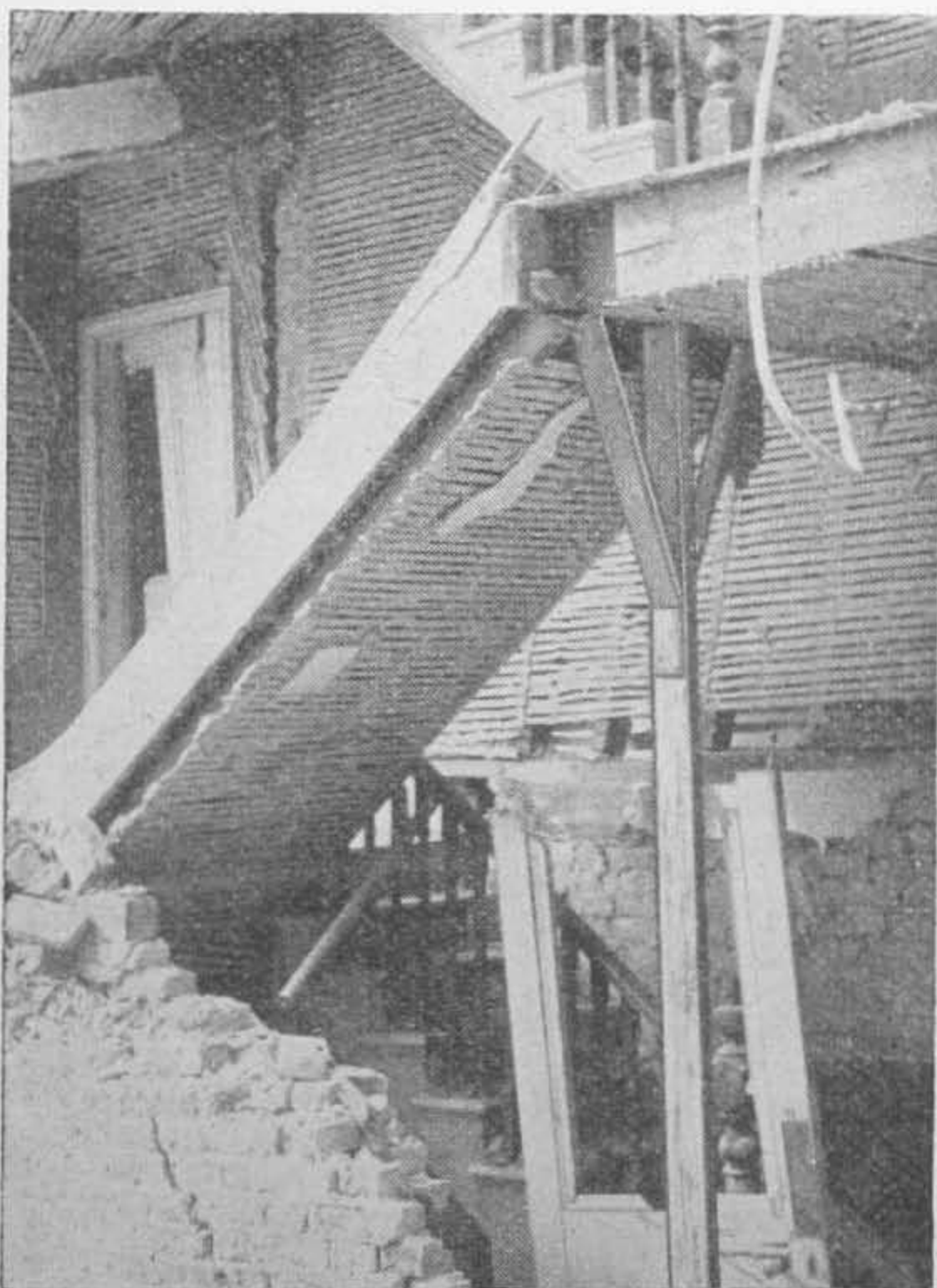
Fig. 125. Temporary shoring showing propping
