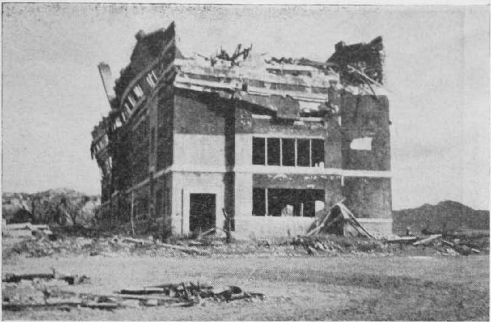
Fig. 5. Further away from ground zero, buildings are pushed over or distorted away from the explosion: Nagasaki, 1945
