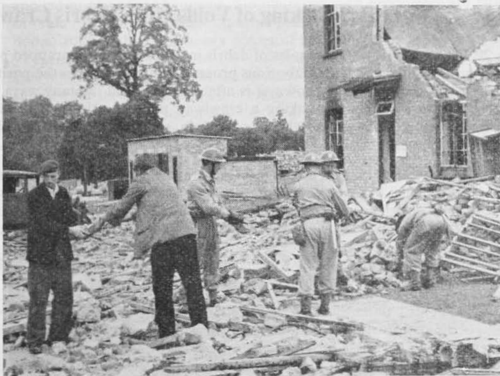
Fig. 82. A human chain for the removal of debris
