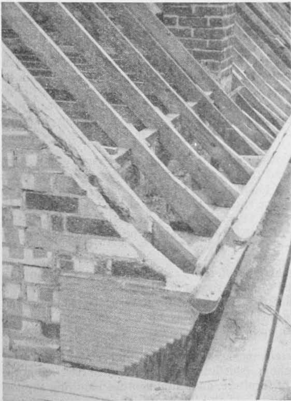
Fig. 15. Details at eaves of roof
