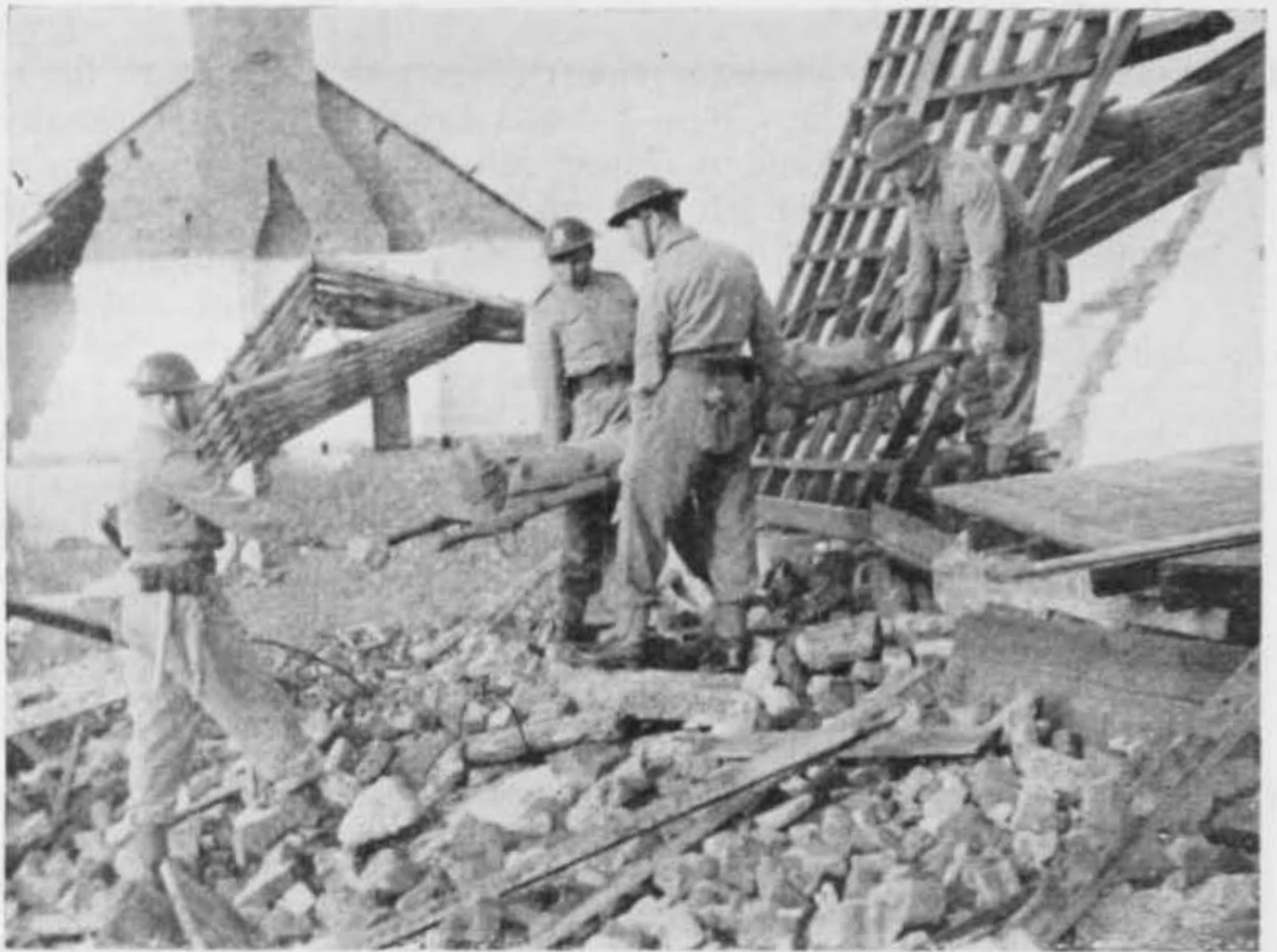
Fig. 35. Moving a stretcher over debris
